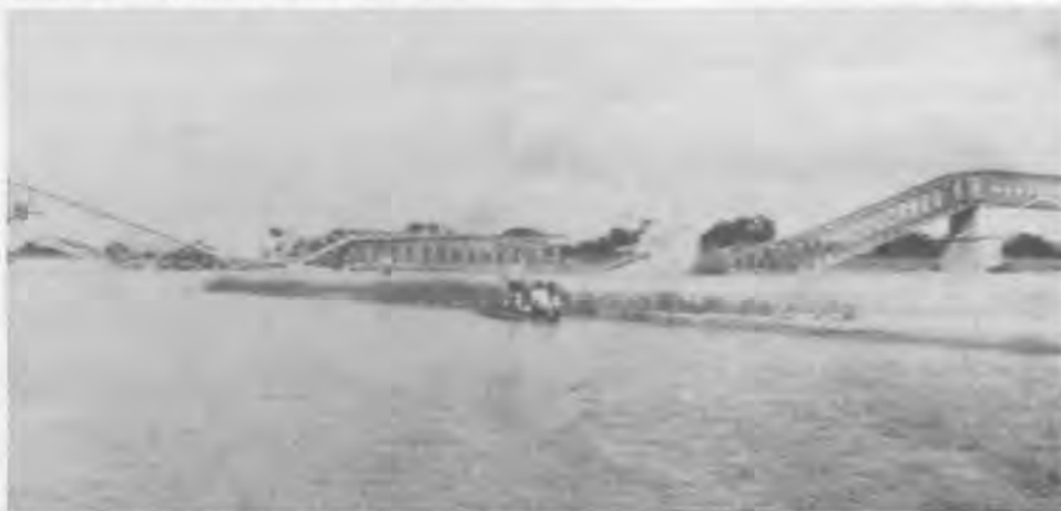
Broken rail bridge, Loire River at Blois, France, bombed by the 466th on 11 June 1944.
