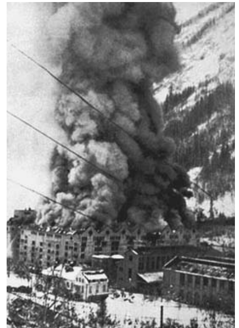
Burning buildings during the 16 November 1943 raid on Norsk-Hydro Vemork plant at Rjukan. PHOTO COURTESY OF NORSK HYDRO ASA.
